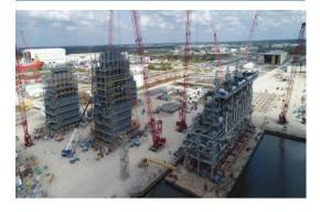
2,900-ton Secondary Quench Exchanger (SQE) module and three 2,500-ton process modules for Ethane Cracker Facility. Offshore Wind Turbine Foundations
