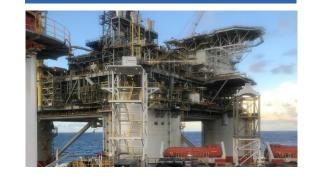
Hookup of a Tension Leg Platform at an offshore location. Facilities are connected to subsea equipment on the ocean floor to allow for hydrocarbon production.
